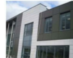
GLAZING CURTAIN WALLING PROFILE
